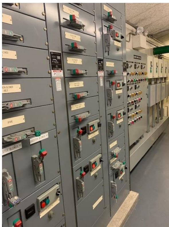
This is the Motor Control Center at the Seal Harbor Treatment Plant, which controls the pumps and aeration blowers for the facility.
