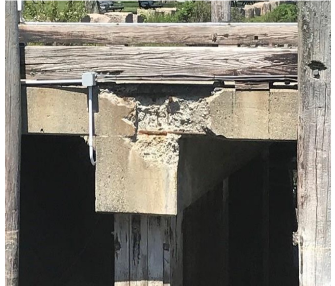
Main pier. Photo shows corrosion of concrete caused by age and salt.
