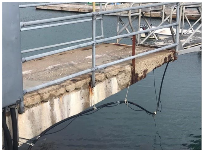
North walkway for access to finger floats. Photo shows corrosion caused by salt corrosion.
