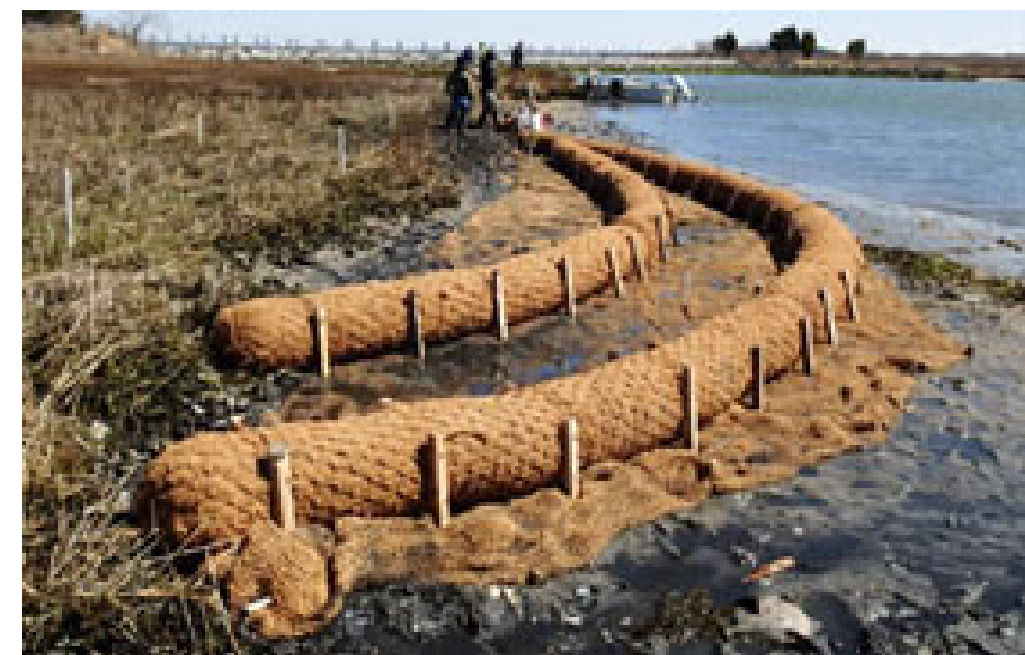
STAKED EXCELSIOR SILT BARRIER
