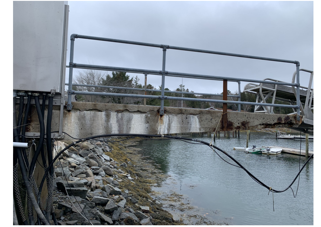
EXISTING FAILING CONCRETE ABUTMENT
