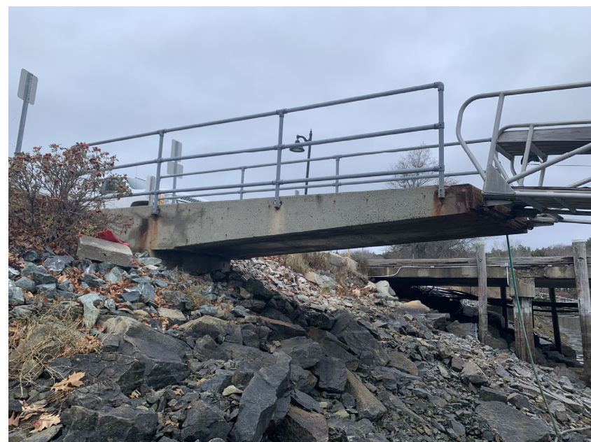
EXISTING FAILING CONCRETE ABUTMENT
