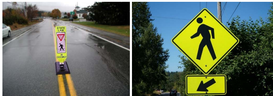
On the left: an example of an in-street pedestrian warning sign (R1-6). On the right: an example of a pedestrian warning sign with arrow plaque (W11-2 and W16-7P).
