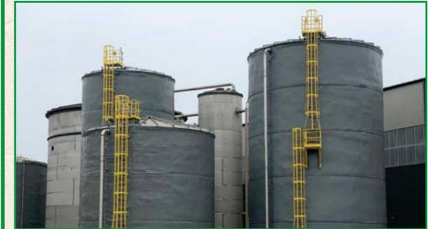
The watery stream of organic wastes, like food leftovers, flow into the anaerobic digester. Like a stomach, this digests the organics into a renewable natural gas, leaving the water clean. The clean water is recycled in a closed loop back into the system. The renewable gas is used to power Coastal, offsetting fossil fuels. In the future, it could also be used locally as a natural gas substitute to lower our community's carbon footprint.
