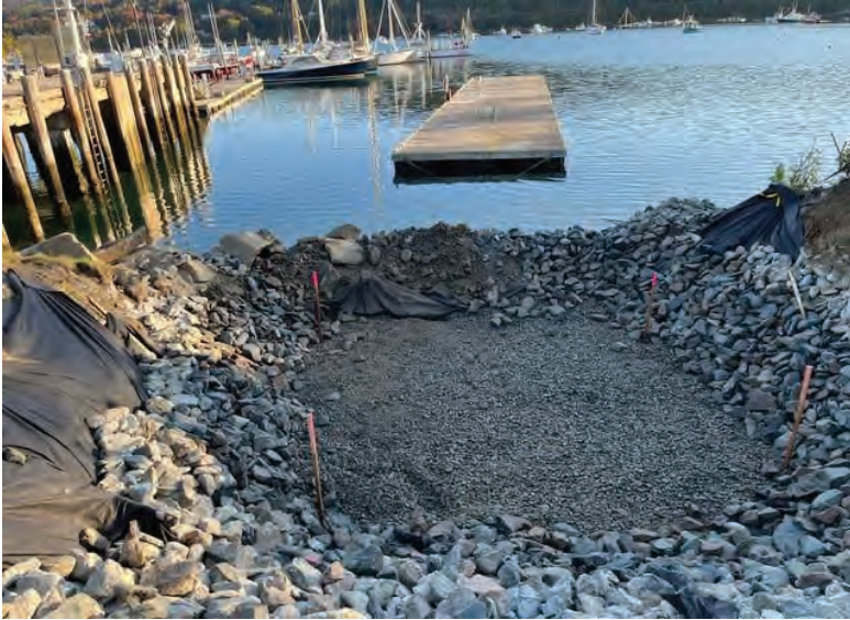
Photo of the south ramp groundwork, preparation for the ramp foundation. October 2022
