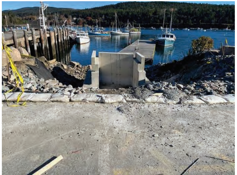
South ramp foundational abutment to support the ramp to the public dock, November 2022
