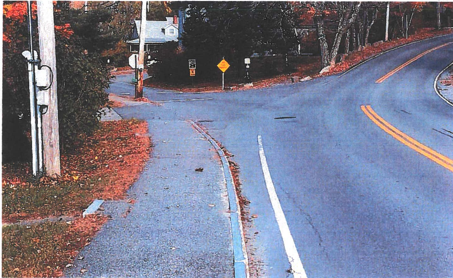
Sewer manhole in RTE#3 towards Jordan Pond Road
