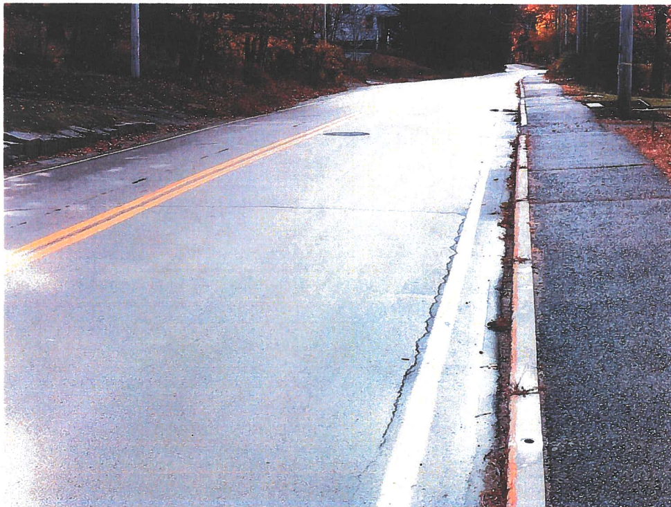
Sewer in Street South towards Steamboat Wharf
