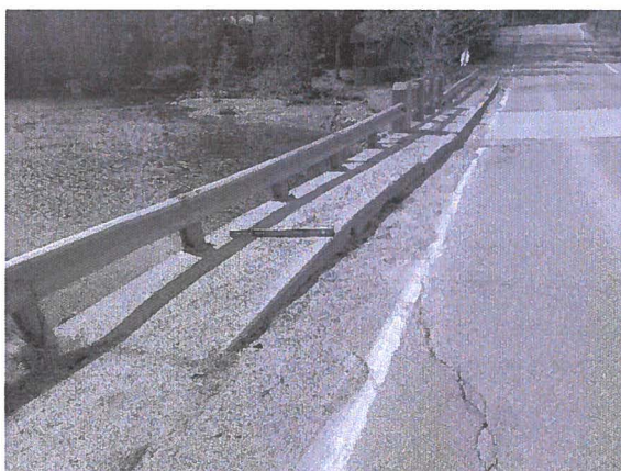
Existing Sidewalk and Ramp
