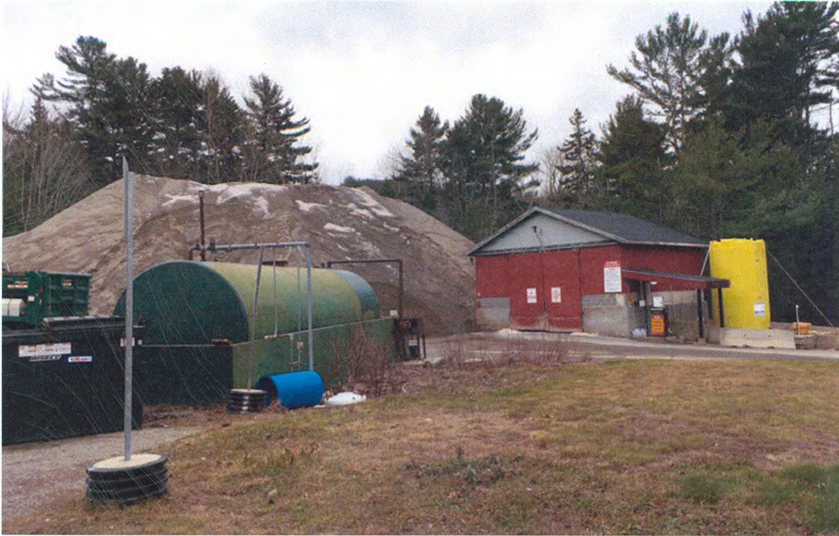
Figure 4. Auxiliary Building and 10,000 Gallon Diesel Tank
