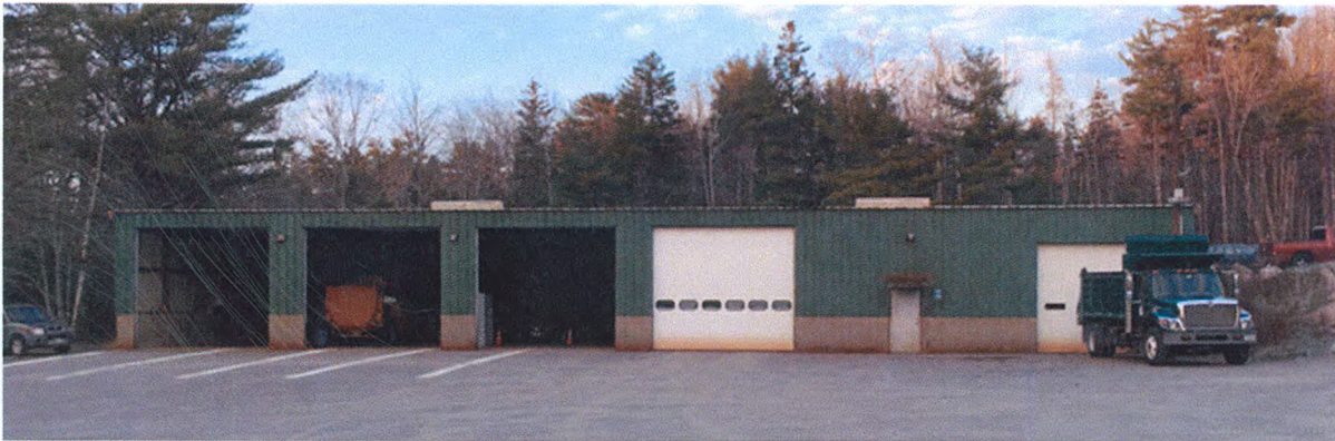
Figure 3. Bus Garage Building
