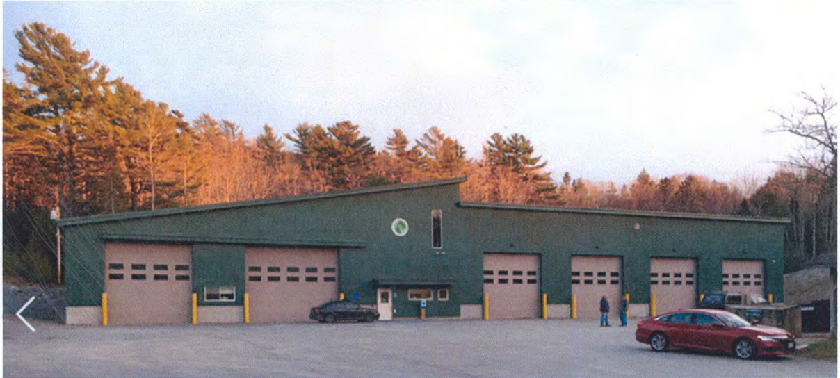
Figure 2. New Municipal Garage Building
