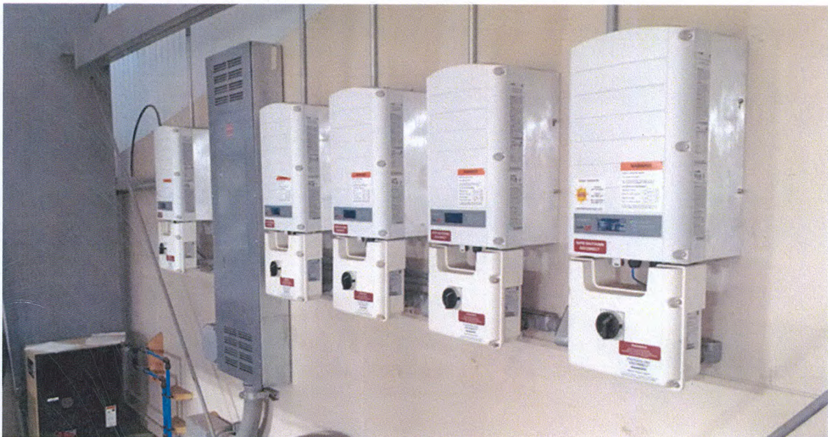
Figure 10. SolarEdge Inverters
