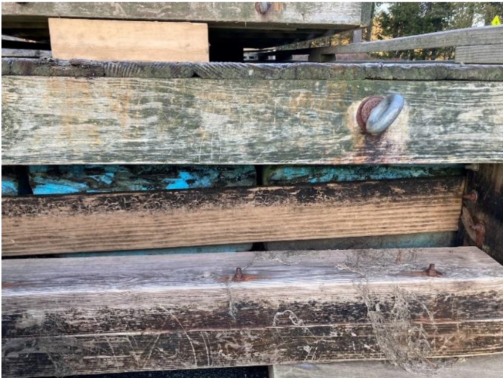
Current dock construction
