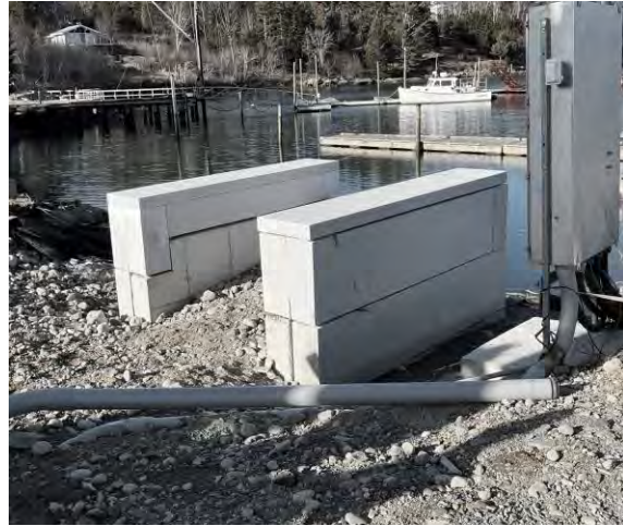
Construction of North Ramp Footings
