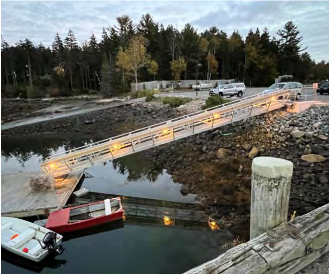
New Public Ramp in Northeast Harbor
