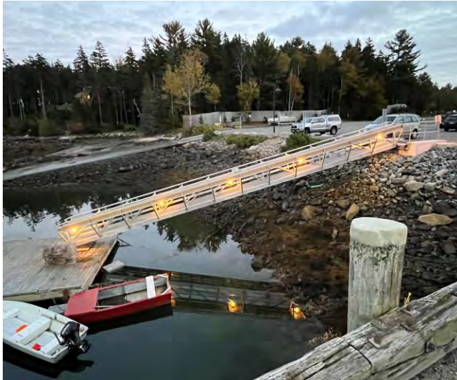
New Public Ramp in Northeast Harbor
