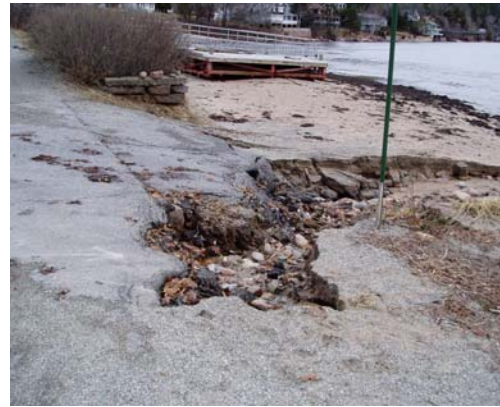
Heavy rains in 2005 washed out the road adjacent to Seal Harbor Beach.
