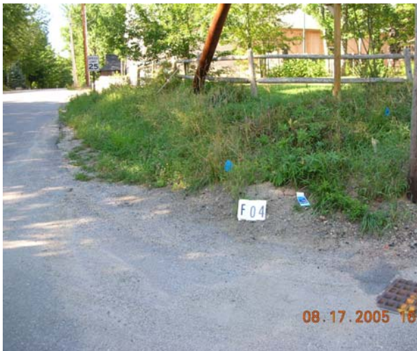
Road shoulder erosion results in sediments flowing directly into storm drains.
