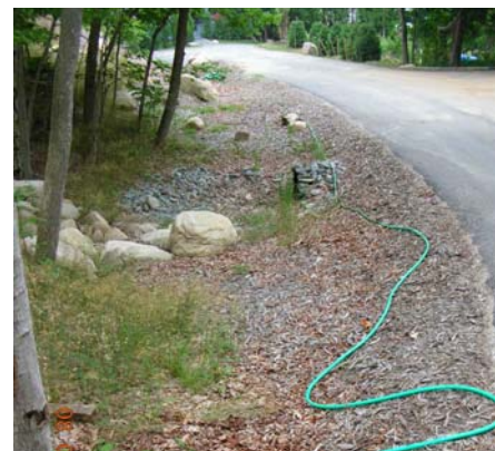
Private road shoulder covered with mulch to prevent shoulder erosion.
