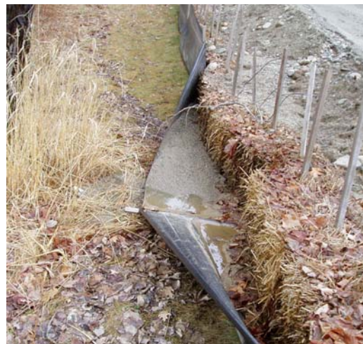
Silt fence and bales of hay failed to contain sediments at this construction site near Stanley Brook.
