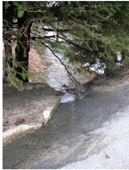
However, this curbing is being used to direct runoff into Stanley Brook.
