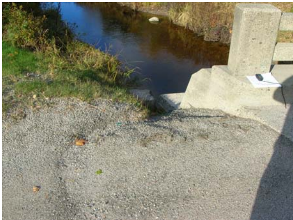
Pavement around the Rte. 3 bridge directs stormwater into Stanley Brook.
