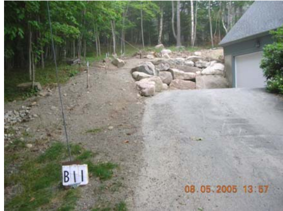
Work around this driveway has disturbed natural vegetation. Soil can be transported in rainwater over the impervious driveway surface.
