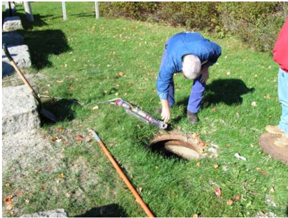
Figure 11: Seeking broken sewer lines: Mt. Desert public works personnel send a camera into the sewer line running beneath Stanley Brook, October 2005
