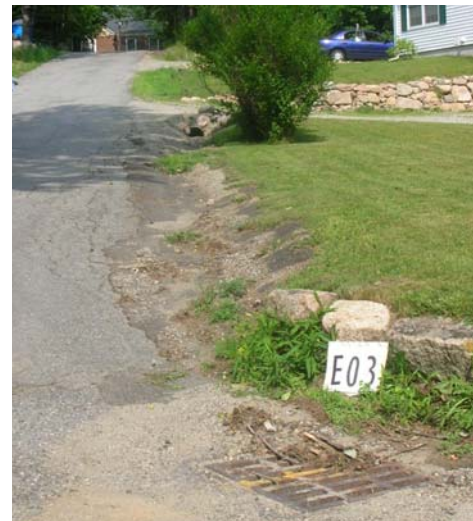
Road shoulder erosion results in sediments flowing directly into storm drains.
